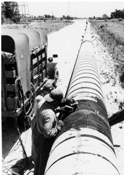
FIGURE 4.44 Pipeline weld MPI using prods.
