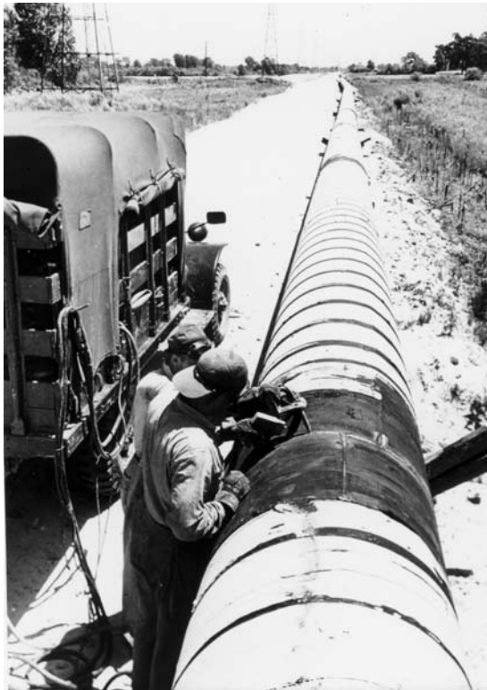
FIGURE 1.6 Magnetic particle inspection of a pipeline weld. (Courtesy Magnaflux.)
